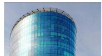
Image: Installed on walls (provided by NEDO)
