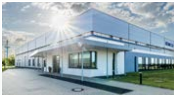
Bautzen DC4 Data Center (Germany)
